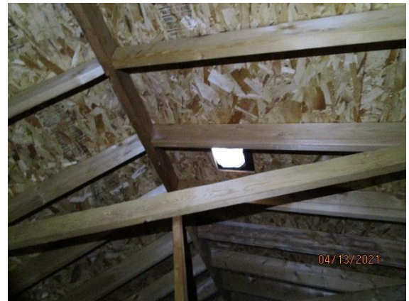
Attic Framing/Sheathing: Roof sheathing with static attic vent
