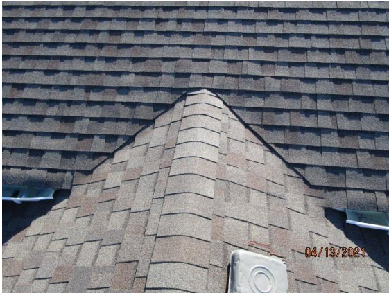
Flashing/Valleys: Junction of upper home to lower home roofing
